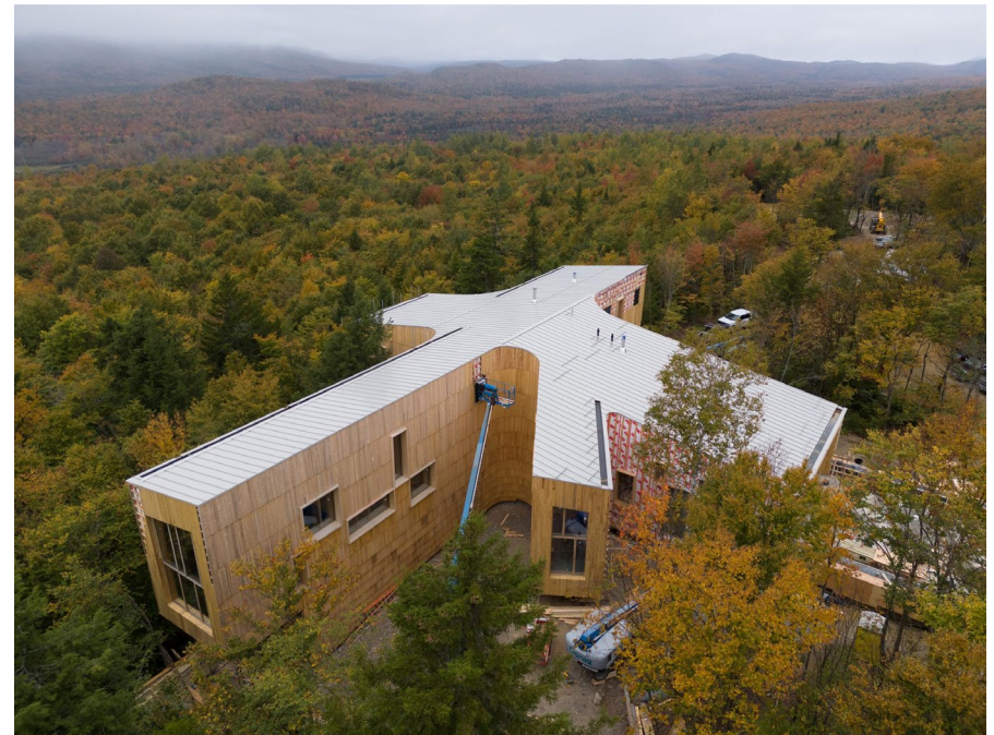
Tekakapimək under construction, Credit: Wright-Ryan Construction
